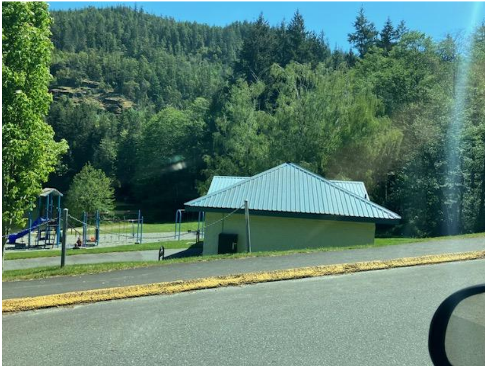
Figure 36. Mowat Bay Park outbuilding with non combustible siding and metal Roof
